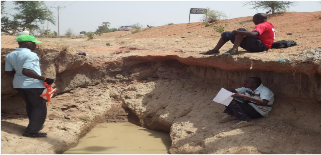
PLATE 1: A typical example of a gully erosion showing an actively migrating headcut in upstream direction at Sangere 6
